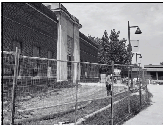
Design and Construction renovating the Old Art Building
