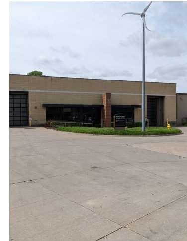
Madison Street Services Building Building 0160
