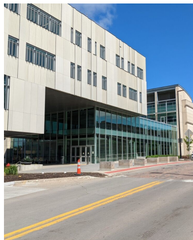
Seamans Center Addition Building 0022
