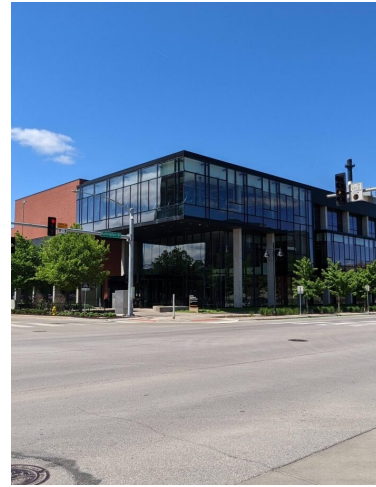
Campus Recreation and Wellness Center Building 0068
