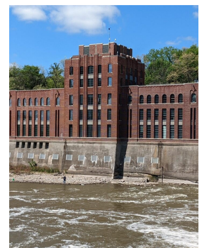
Stanley Hydraulics Lab Building 0024
