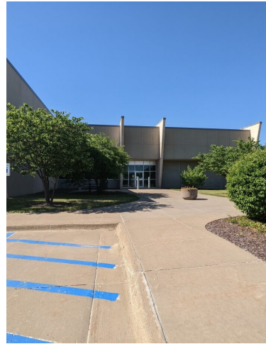
Information Technology Facility Building 0290
