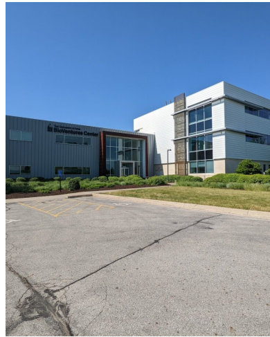
Bioventures Center Building 063
