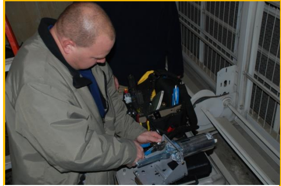
Photo: Energy Hawk Scott Sellner repairs an actuator in the Lindquist building.
