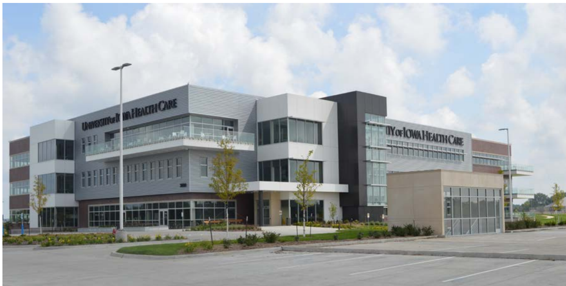
Health Care Support Services Building
