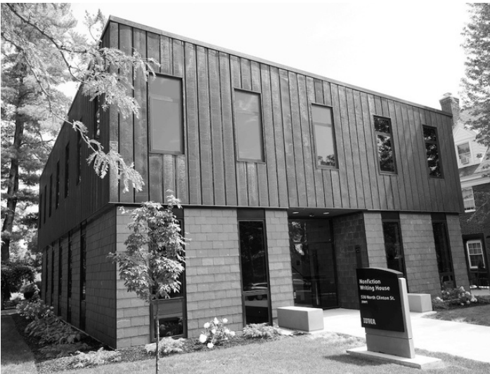
The newly-completed Nonfiction Writing House on the corner of North Clinton Street and Church Street
