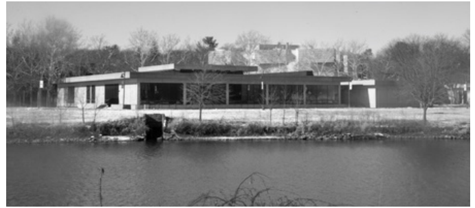
The Performing Arts Annex that will be renovated to house the Department of Dance
