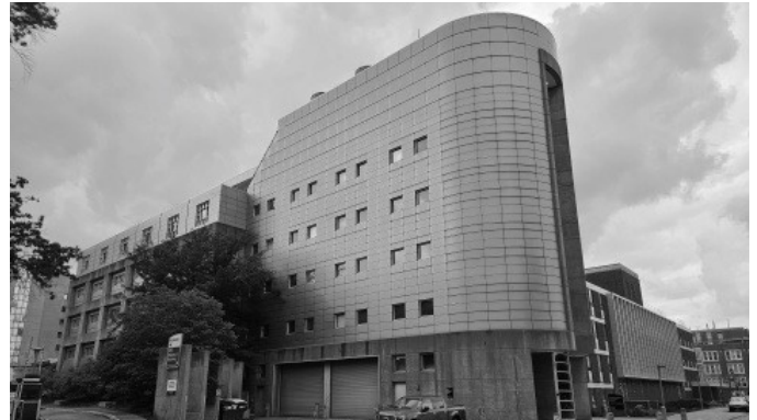
The newly-named Iowa Bioscience Innovation Facility, formerly the College of Pharmacy
